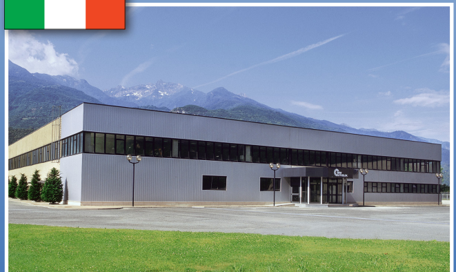
AUTOBLOK plant Caprie-Torino
